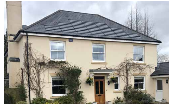
Figure 48: Use of shingle-like solar panels on a slate roof, with the design and colour of the solar panels matching those of the adjacent slate tiles.
